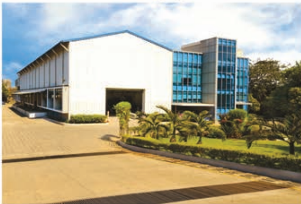
Rainwater Harvesting Tank Below Front Lawn - Unit 1 Vasai
